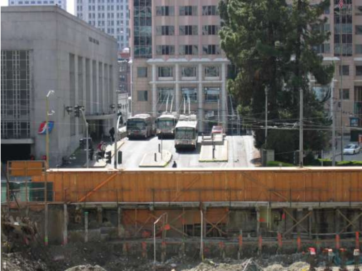
Figure 15 Picture of vehicles on the old Transbay terminal
