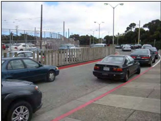
Figure 34: Lack of ADA curb ramp from kiss-and-ride to South Geneva Transit Plaza
