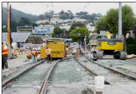
Track Replacement near West Portal Station
