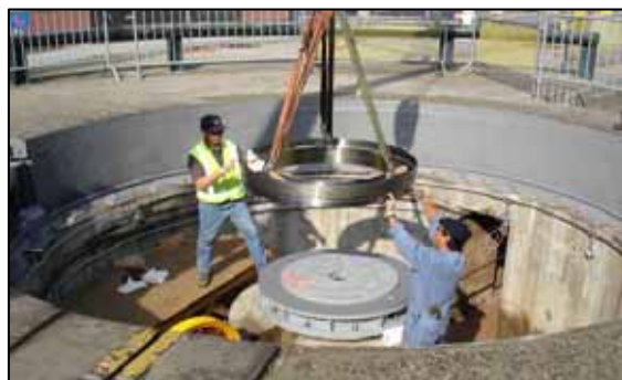
Cable Car Turnaround Work
