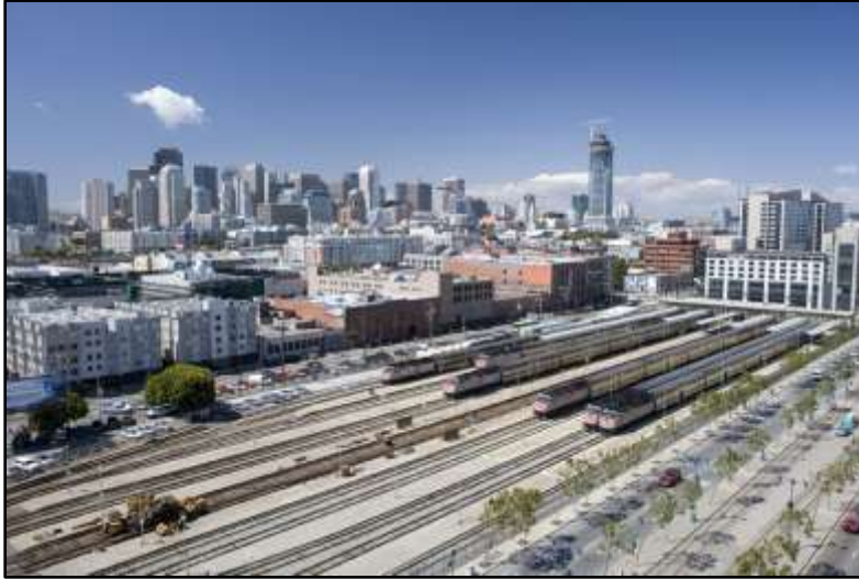
Image: Caltrain station at 4 th and King Streets; photo credit: San Francisco Redevelopment Agency
