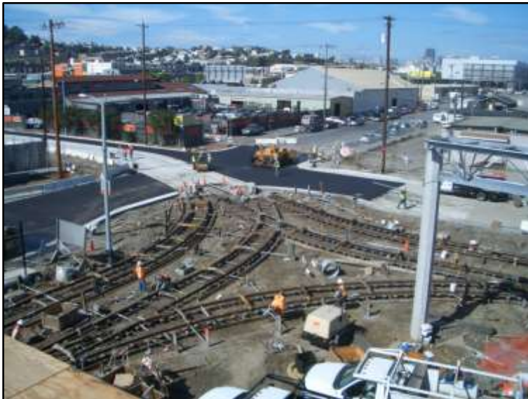
Image: Rail replacement project in progress.
