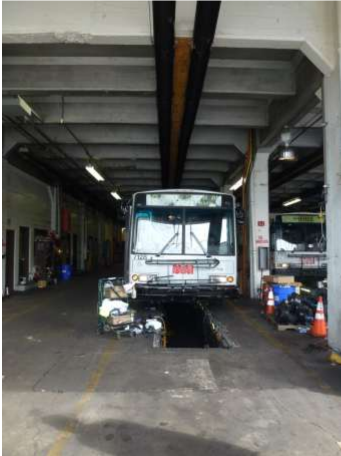
Building height at Potrero does not allow for lifting buses.
