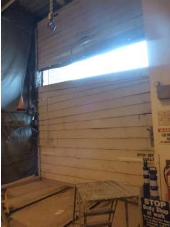
Body shop bay door is broken and leaves the shop open to the elements.
