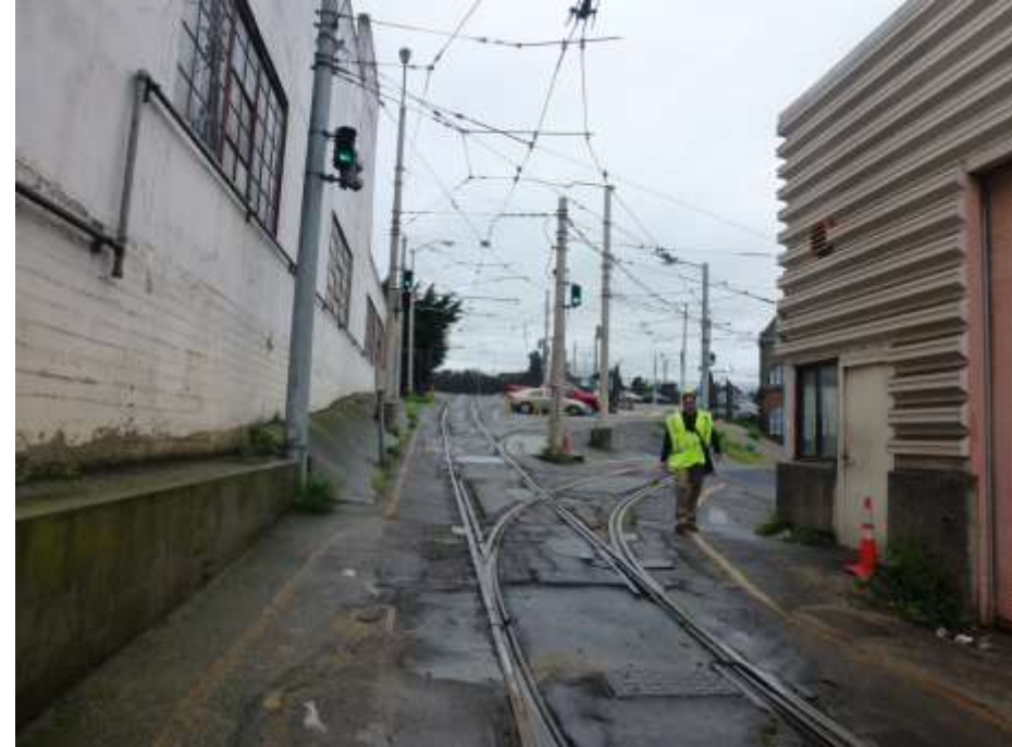
Track turns at Cameron Beach need to be assessed for turn radius.
