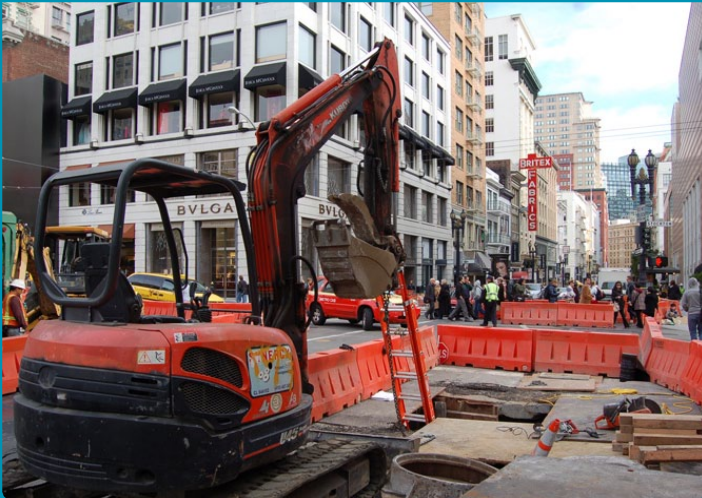
Examples of utility relocation work around Union Square.
