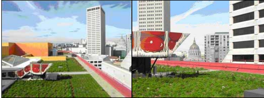
Images: Green roof on SFMTA Headquarters at One South Van Ness Avenue
