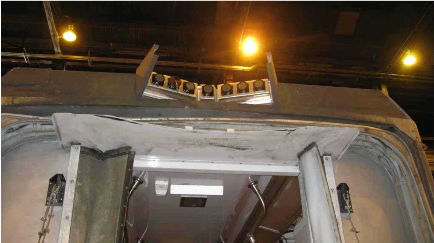
NEWLY INSTALLED CONNECTORS IN ARTICULATION SECTION
