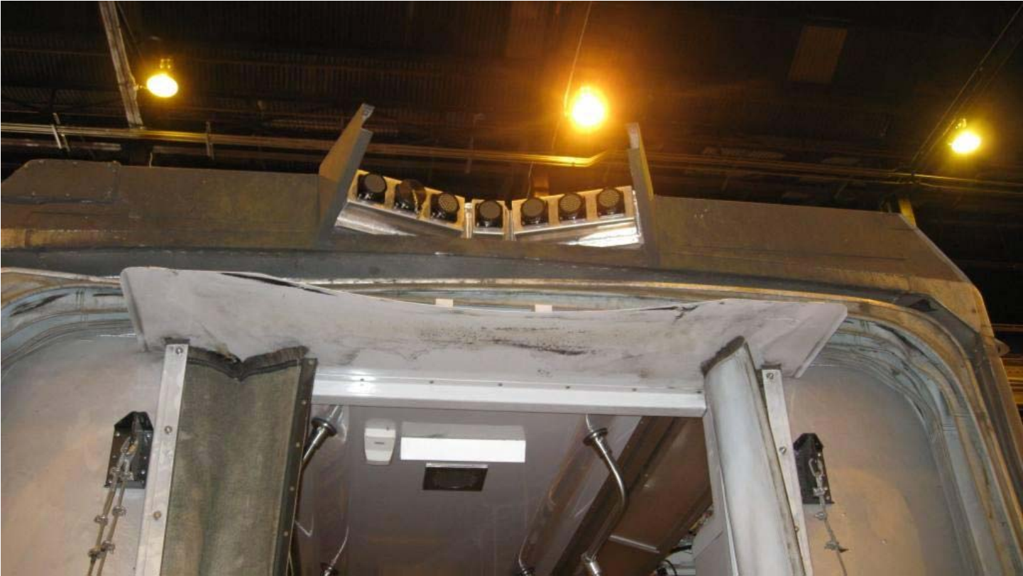
NEWLY INSTALLED CONNECTORS IN ARTICULATION SECTION
