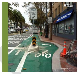
**After:** The SFMTA installed a bicycle signal and an innovative "bike bay" that allows people on bicycle to turn onto southbound Valencia Street via a protected crossing. This improvement closed a crucial gap in the bicycle network.
